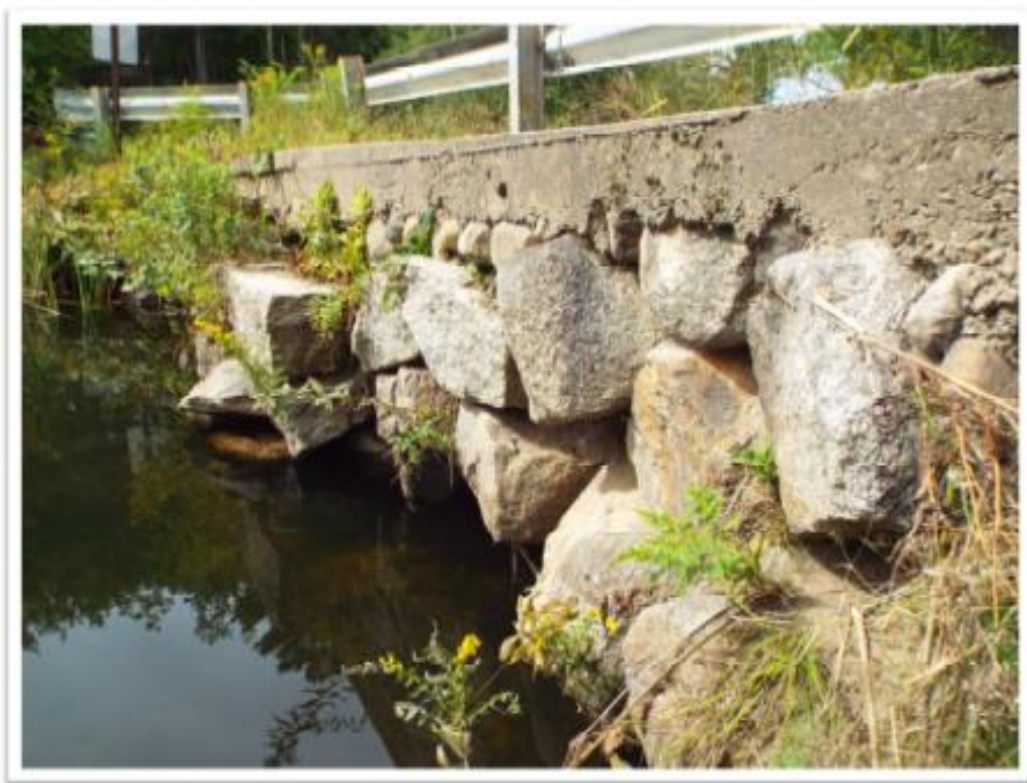
Bailey Road, Effingham –Culvert at Province Lake Outlet
