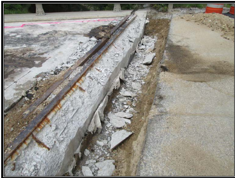
Photo 3: Excavation and demolition at backwall.
