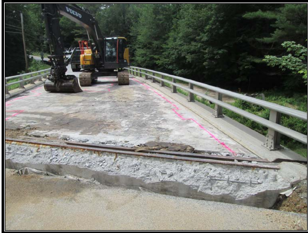
Photo 2: Marked locations for deck repair along the west curb line.
