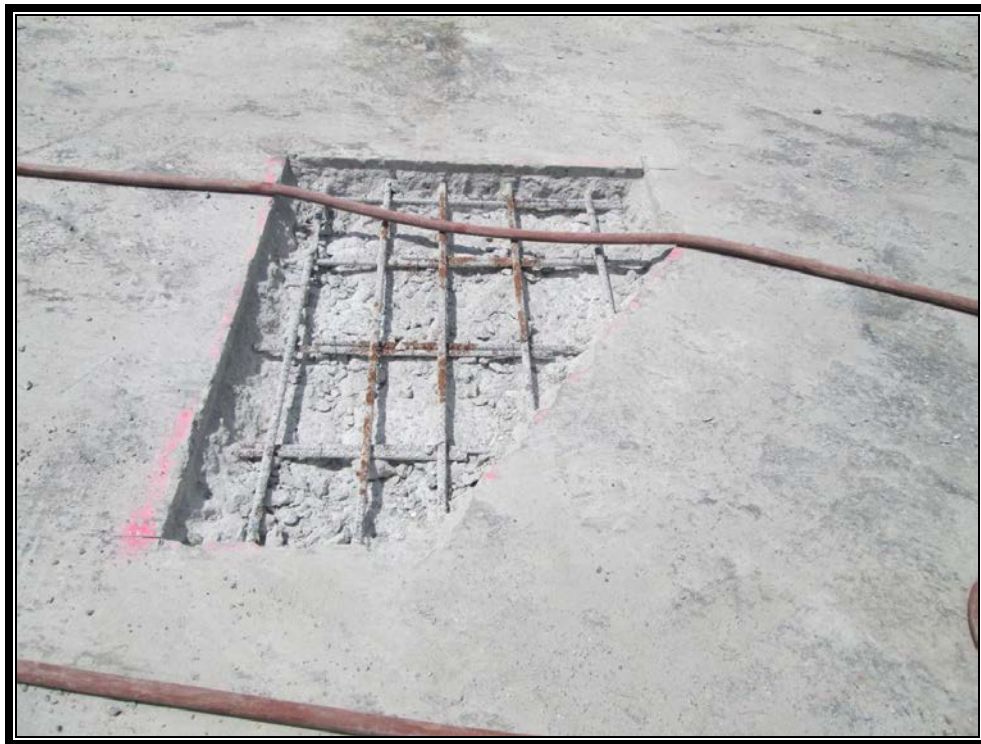
Photo 3: Partial depth repair in middle of deck.
