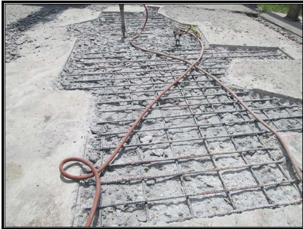
Photo 1: Partial depth repairs in the middle of the deck.
