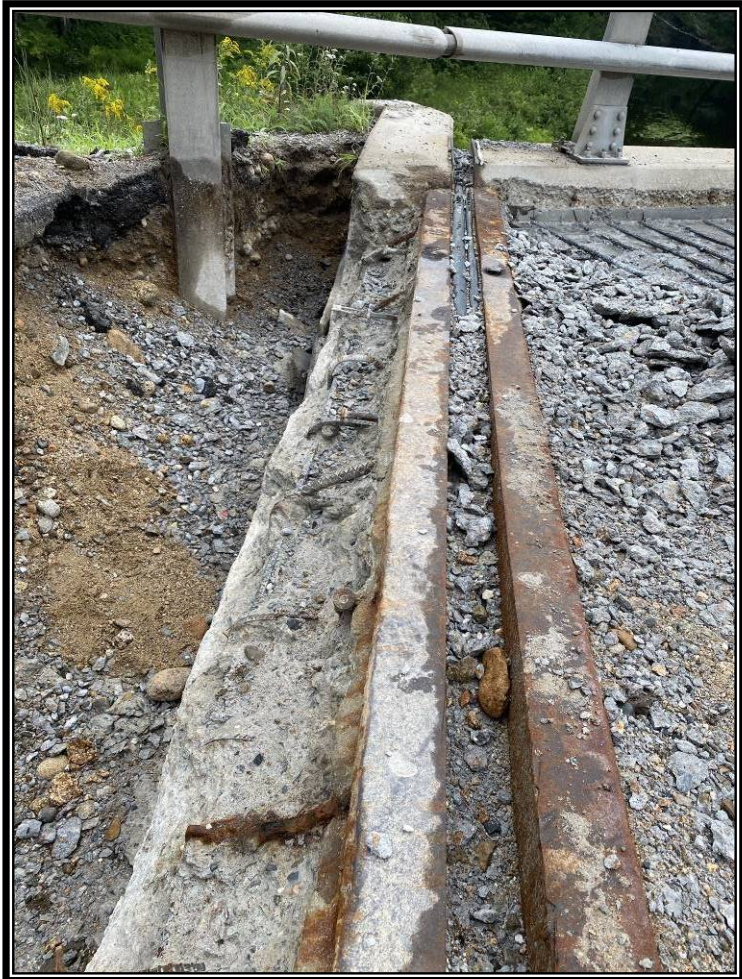
Photo 3: Expansion joint and backwall.
