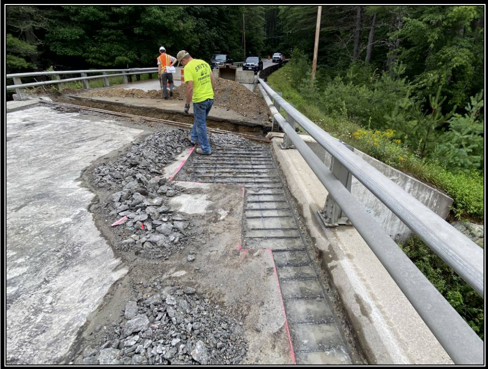
Photo 2: Deck along the east curb prepared for partial depth repairs.
