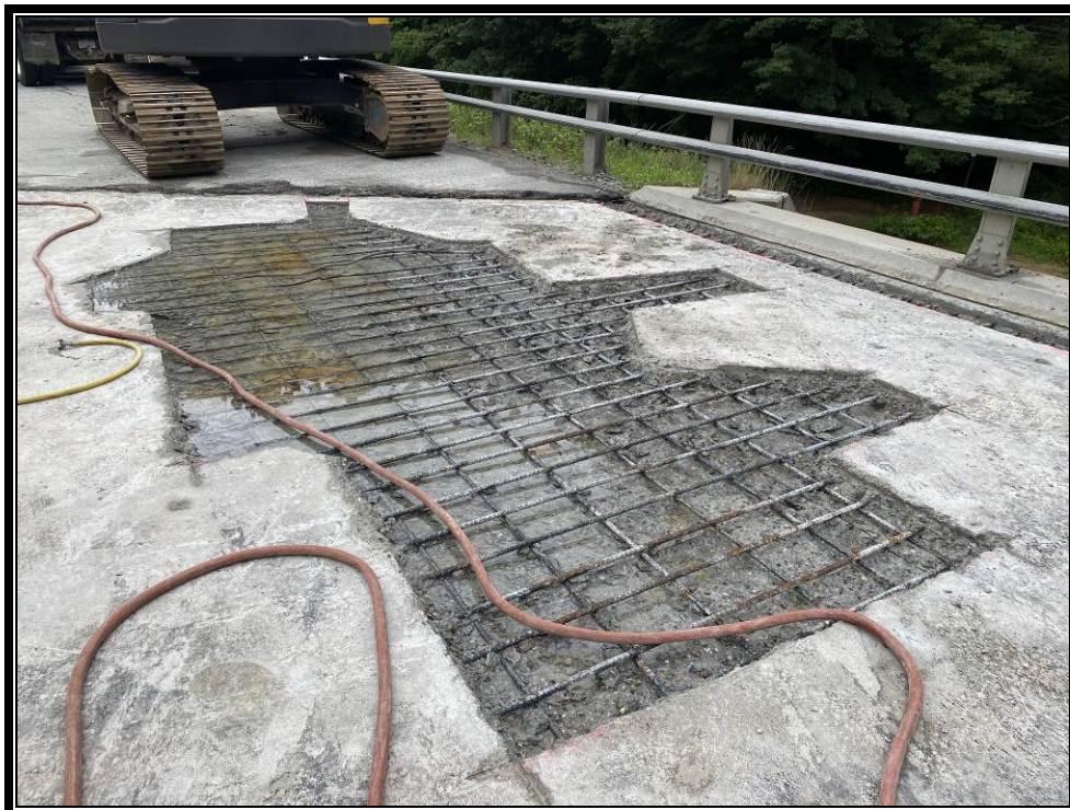
Photo 1: Deck along the east curb prepared for partial depth repairs.
