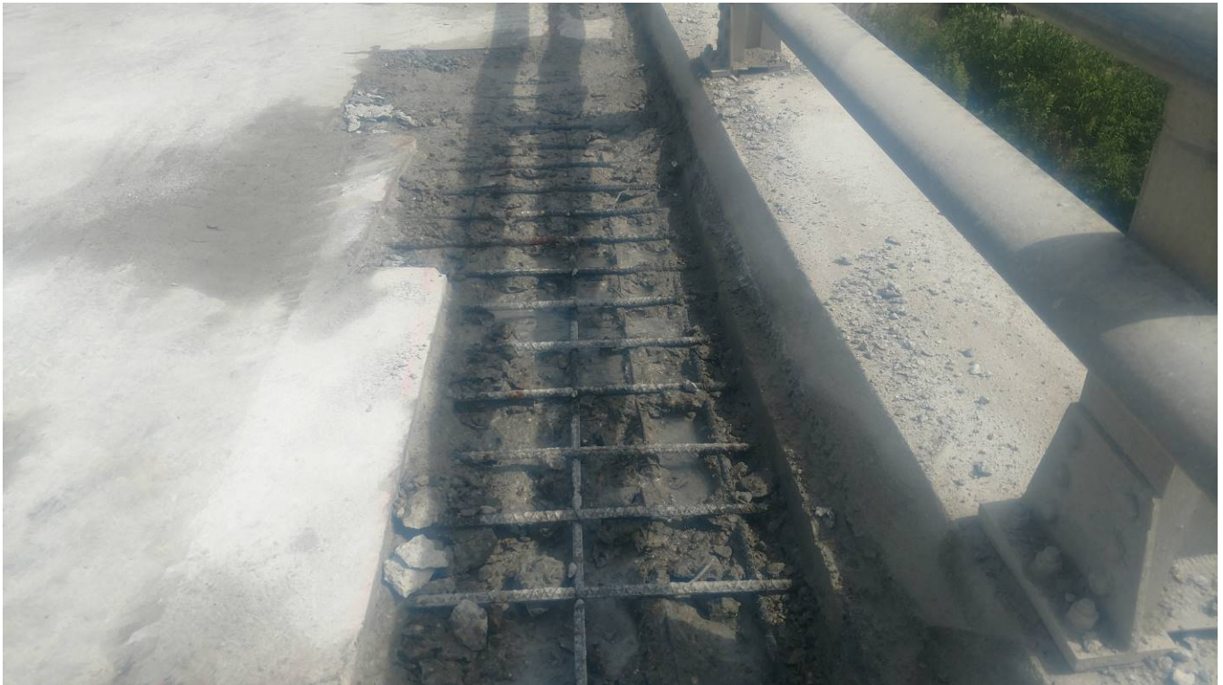
Photo 1: Deck along the east curb prepared for partial depth repairs.
