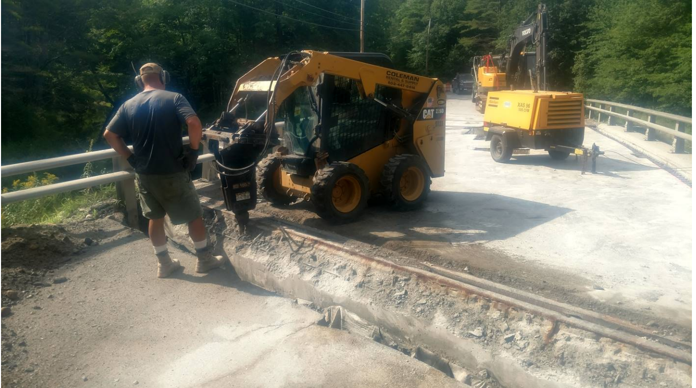
Photo 2: Skid-steer with hammer at the bridge backwall.
