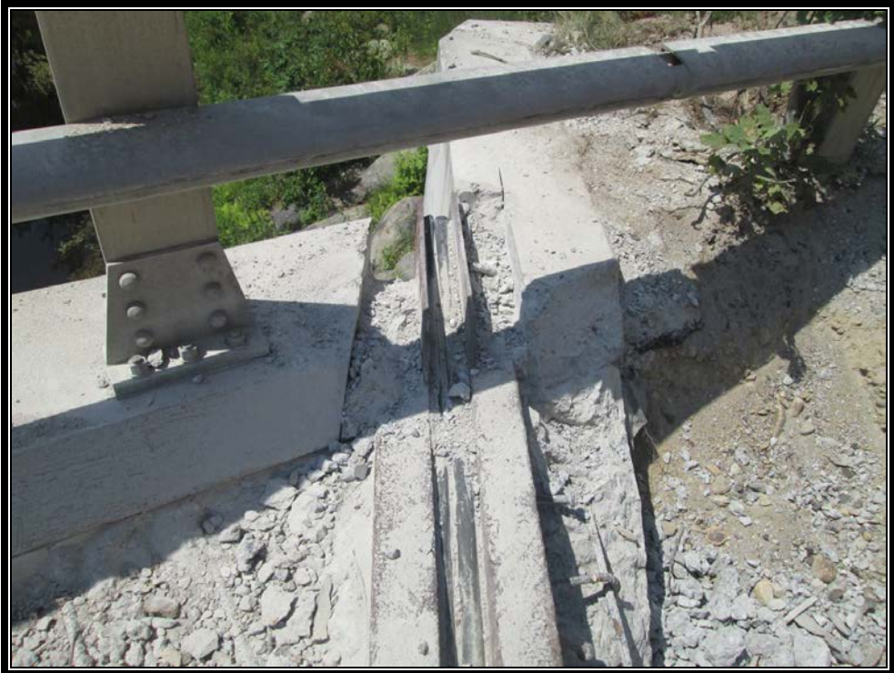
Photo 3: Sawcut and demolition at the curb.
