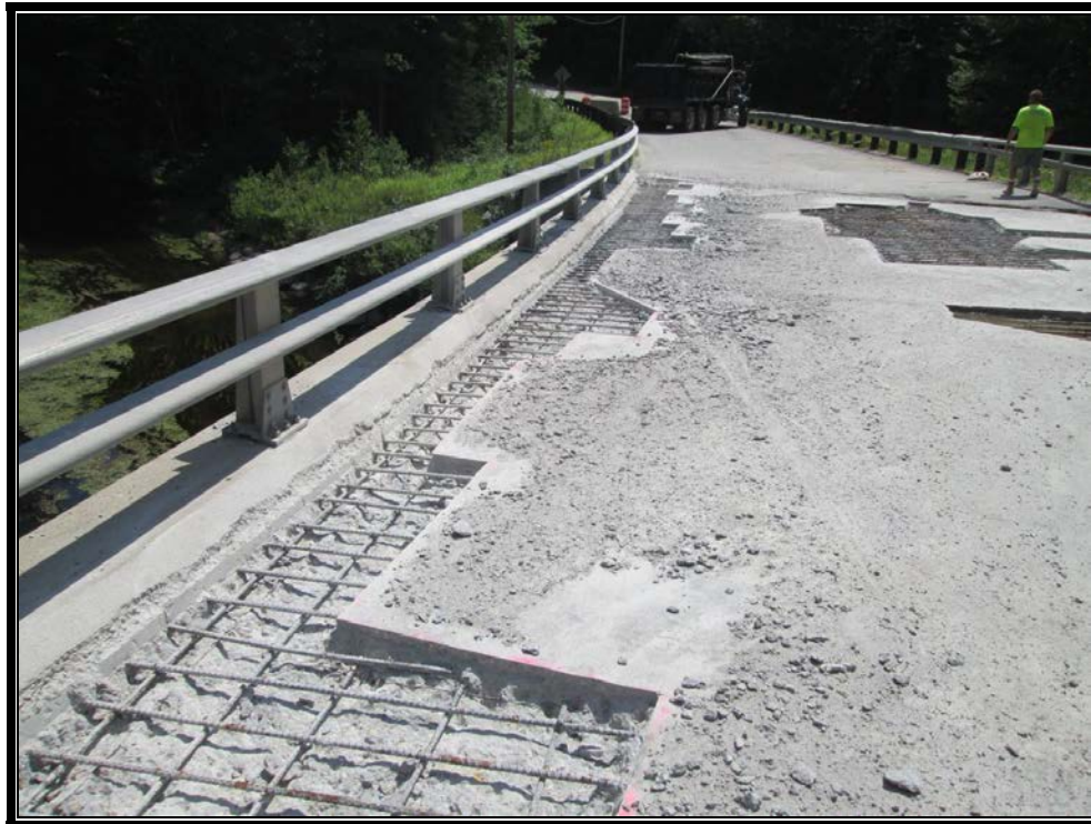
Photo 1: Concrete removed along the east curb.
