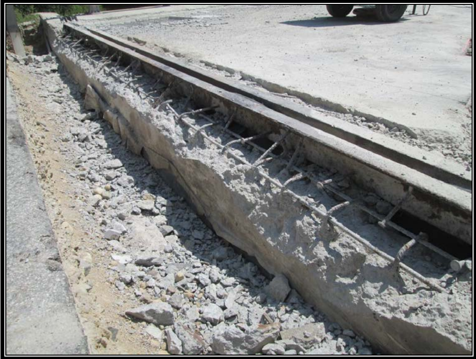
Photo 2: Backwall chipped out to remove the expansion joint.
