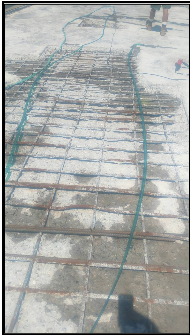
Photo 1: Reinforcing steel spliced into existing steel.
