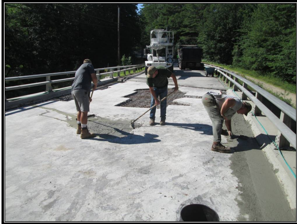
Photo 2: View of crew raking and consolidating concrete.
