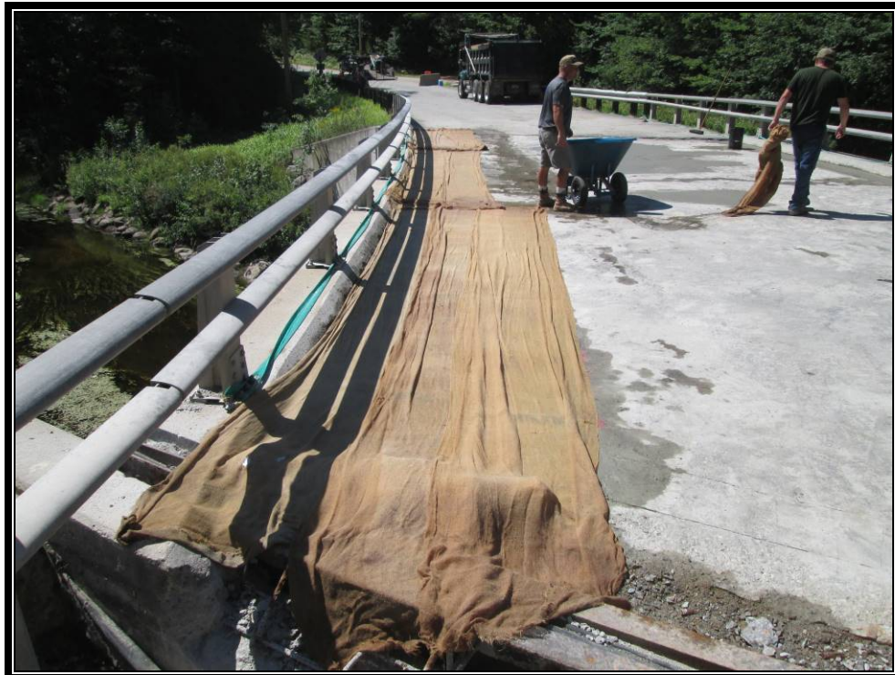
Photo 3: View of wet burlap placed over concrete.
