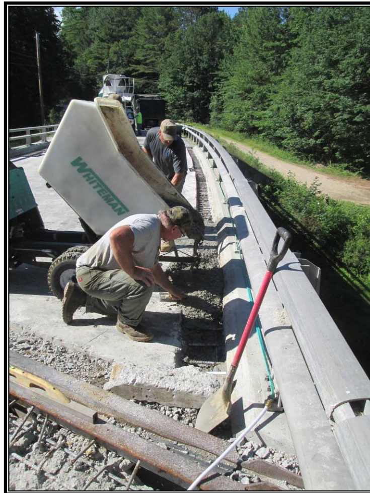
Photo 1: View of concrete from wheelbarrow.
