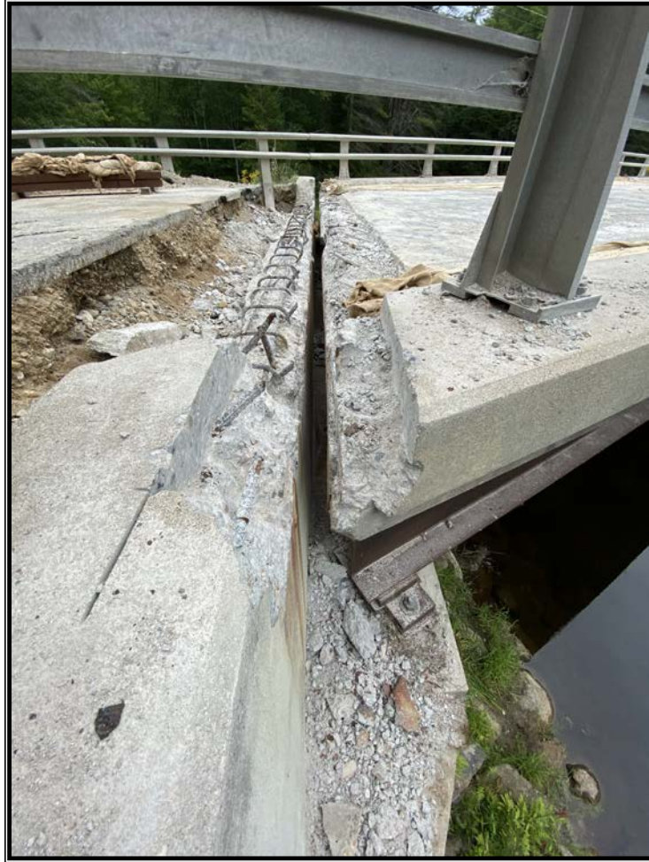
Photo 1: View of deck end and backwall after removal of expansion joint.
