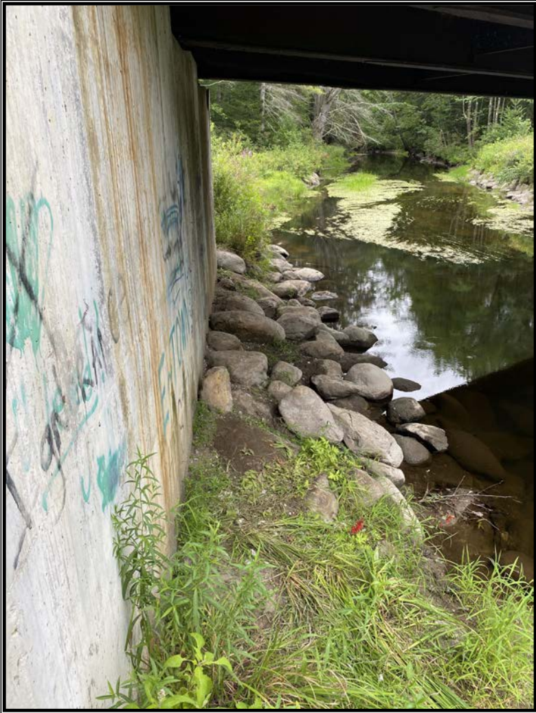
Photo 2: View of river bank after demolition debris was removed.
