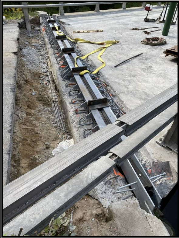
Photo 2: View of expansion joint dry fit.
