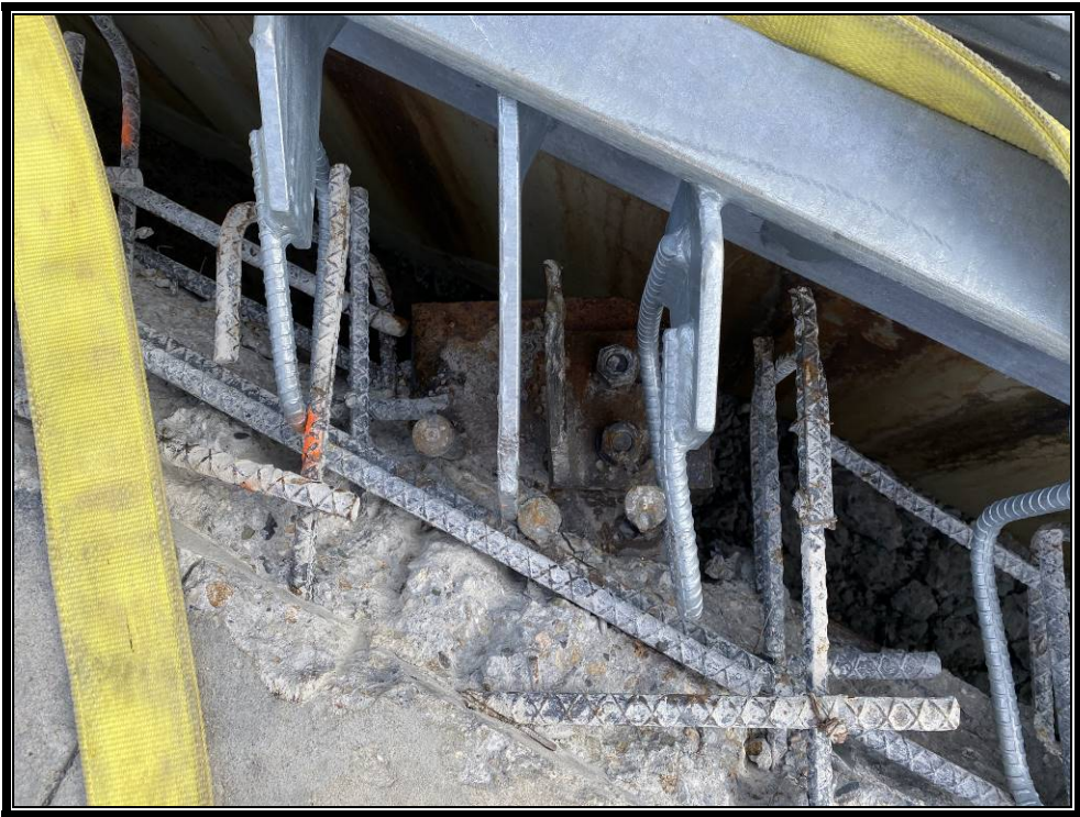
Photo 3: View of joints and connector plates.
