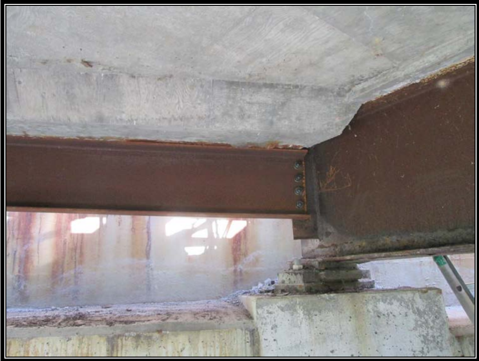
Photo 3: New diaphragm installed.
