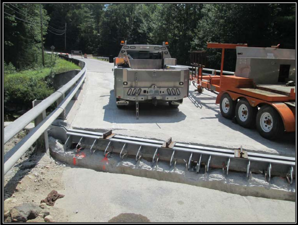
Photo 2: Expansion joint in place with new anchor rods into backwall.
