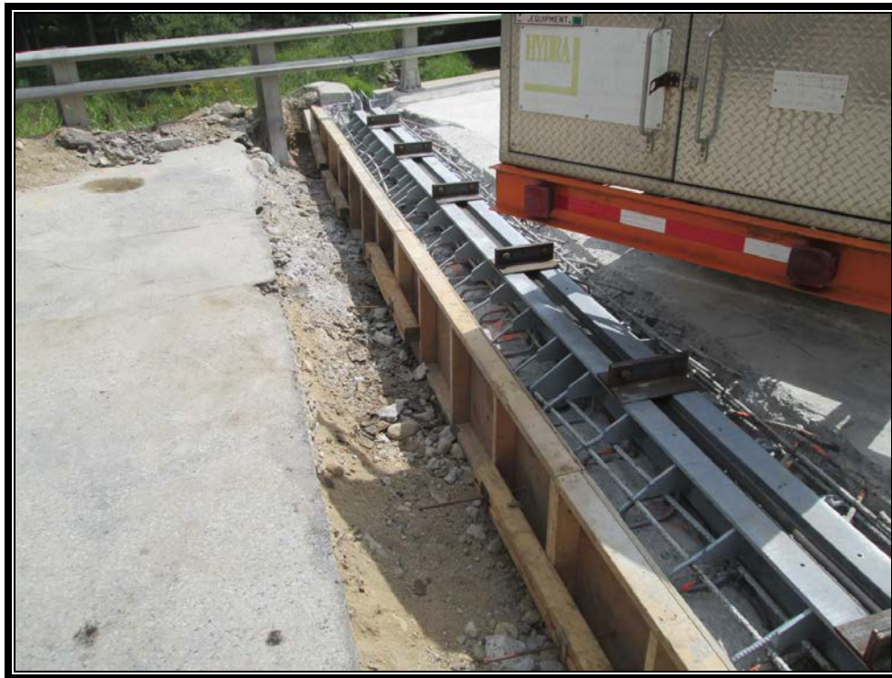
Photo 1: Form installed at backwall.
