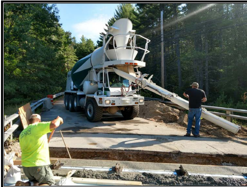
Photo 1: Contractor preparing to place concrete.
