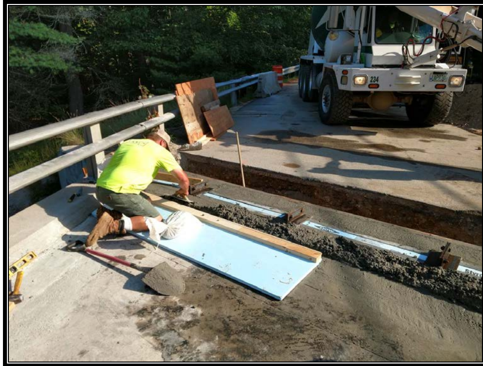
Photo 2: Contractor finishing the end of deck concrete.
