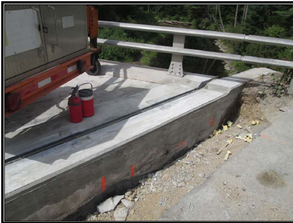
Photo 1: Backwall with forms removed.
