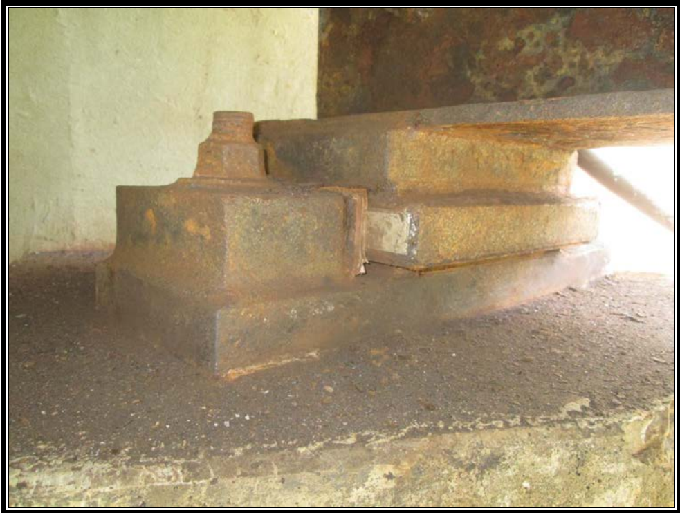
Photo 2: Bridge bearings with loose rust removed.
