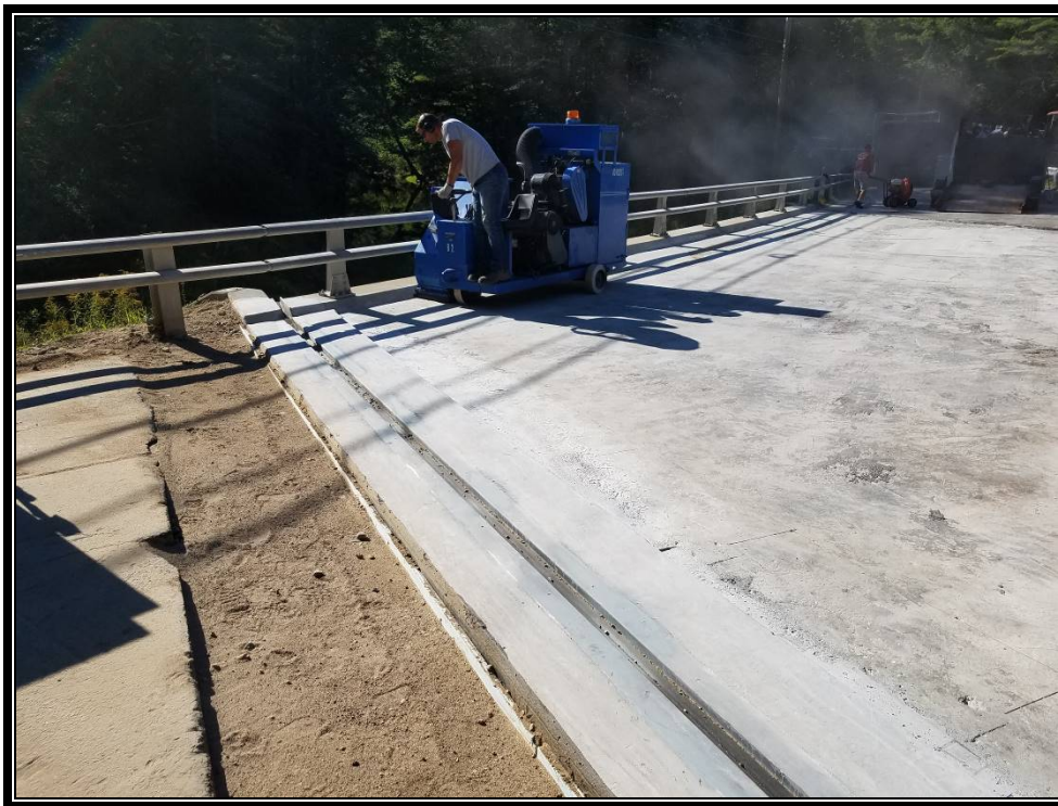
Photo 1: Bead-blasting the bridge-deck.
