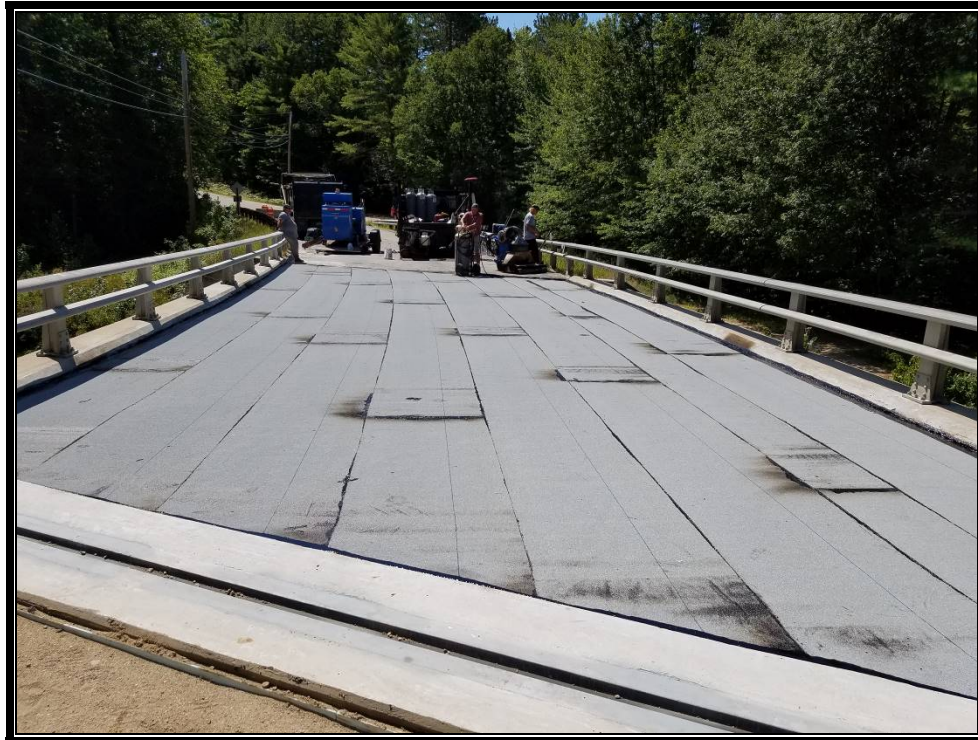
Photo 5: Finished membrane installation.
