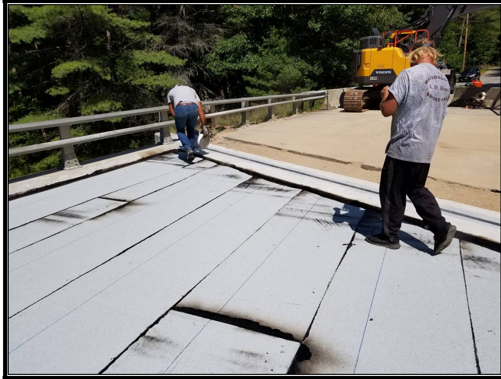
Photo 4: Sealing edges of membrane.
