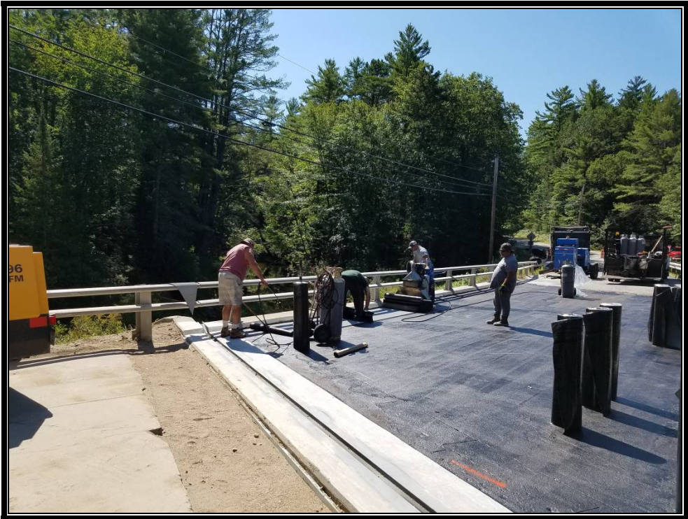
Photo 3: Installing the first row of barrier membrane.
