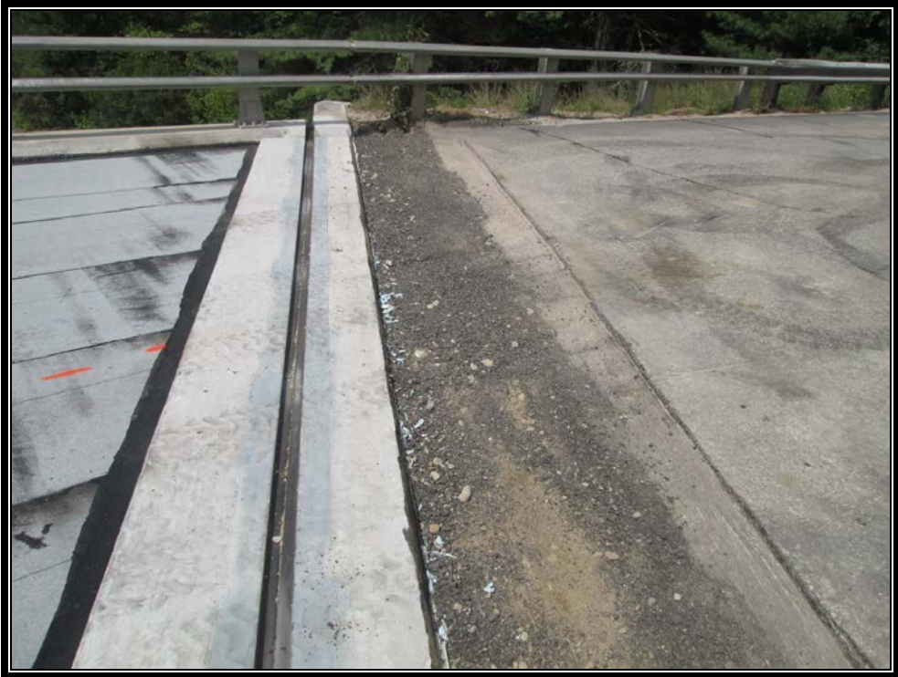
Photo 2: Milled pavement at north approach.
