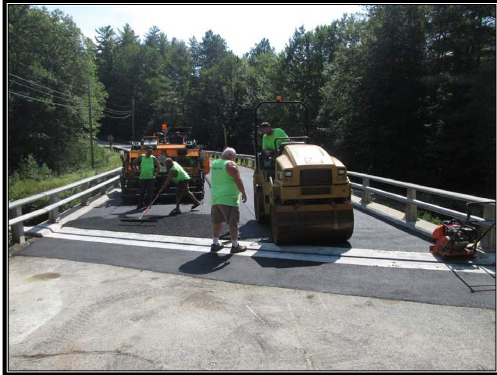
Photo 5: Compacting wearing course.
