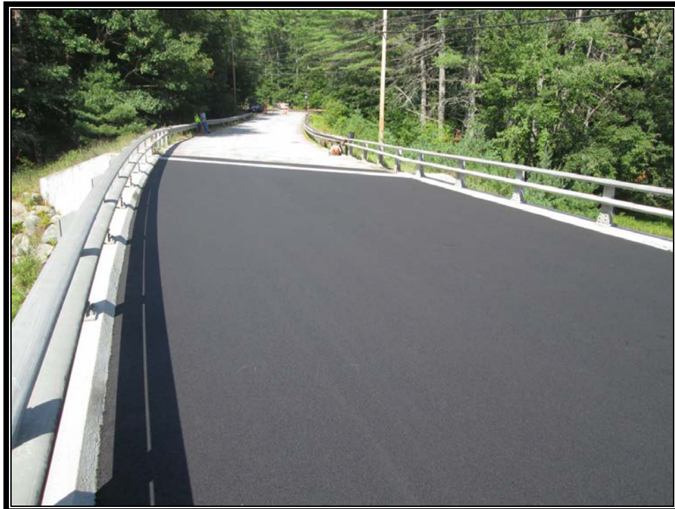
Photo 6: Finished pavement on bridge deck.
