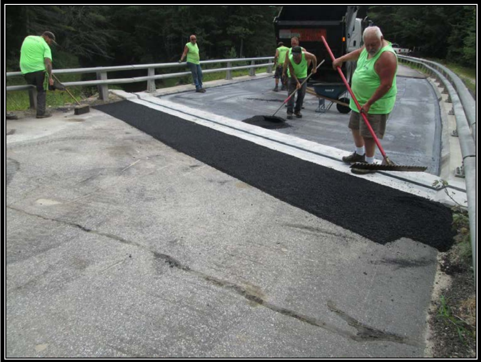
Photo 3: Hand paving at north approach.
