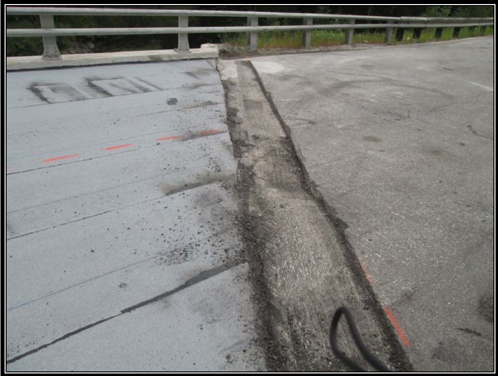
Photo 1: Milled pavement at south approach.
