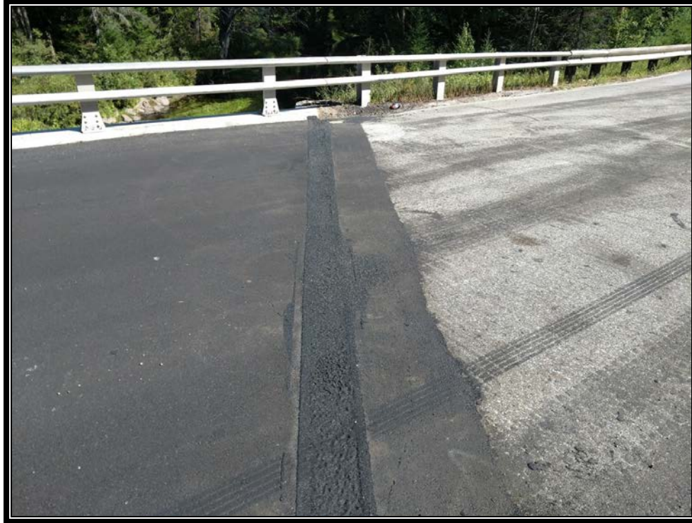
Photo 3: Asphaltic plug joint.
