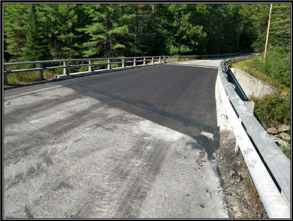
Photo 1: Bridge open to traffic.
