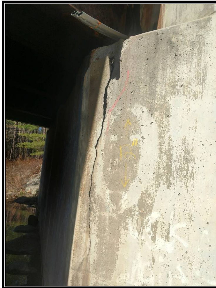
Photo 1: Area of repair at the northeast corner of the abutment.
