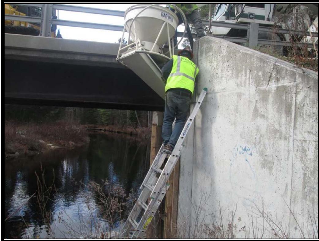
Photo 2: Contractor placing concrete in forms from the bucket.
