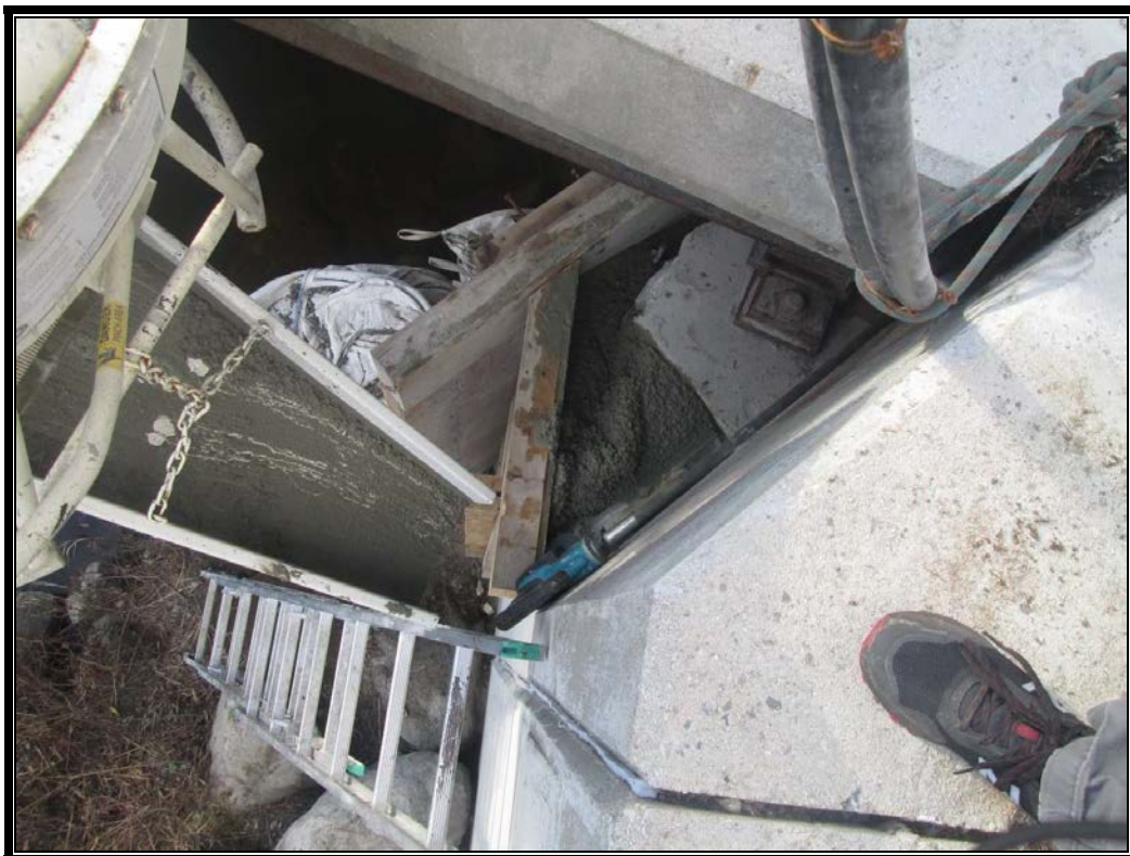
Photo 3: Concrete in forms prior to finishing surface.
