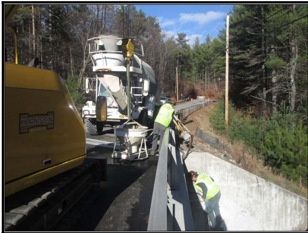
Photo 1: Truck placing concrete in bucket.
