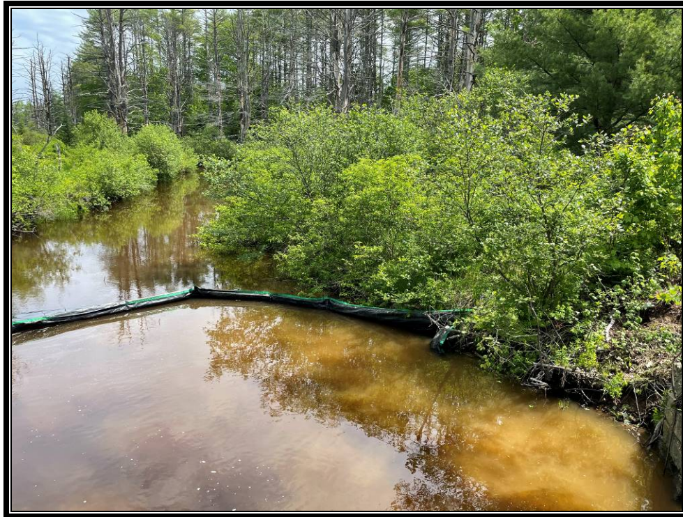
Photo 1: Turbidity curtain downstream of the culverts.
