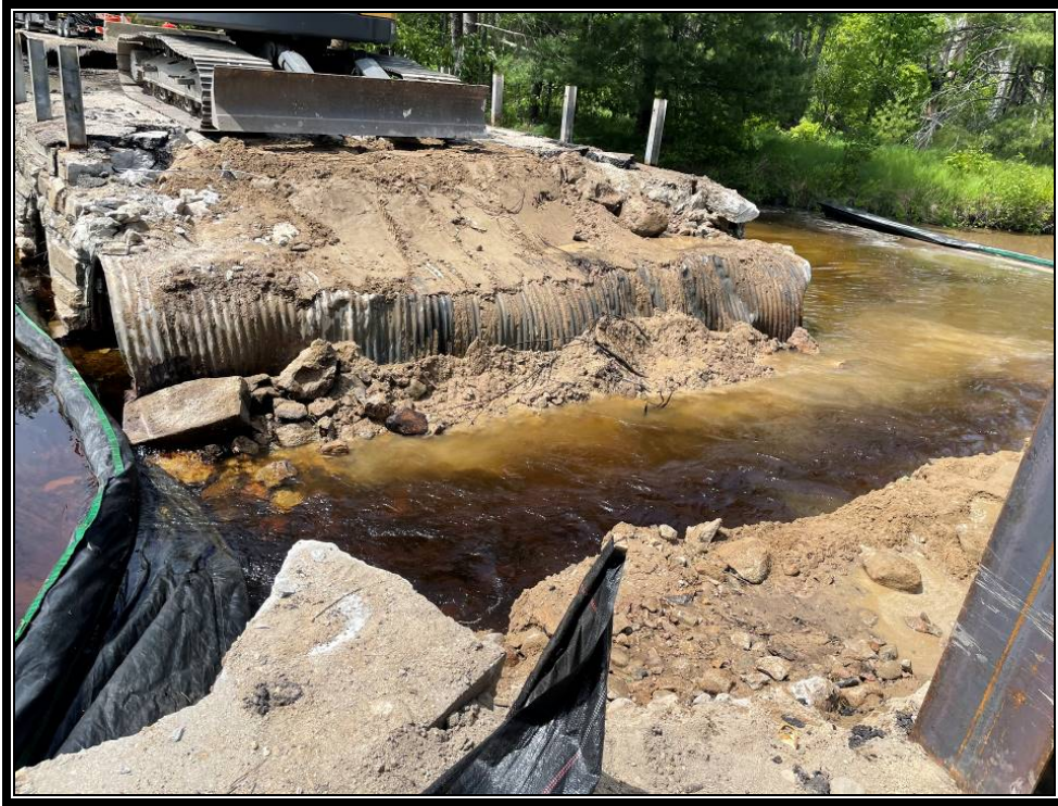
Photo 2: The channel created by removing the culvert.
