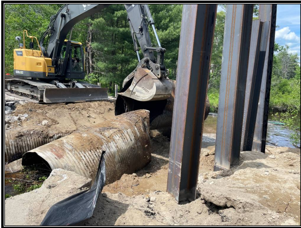
Photo 1: Removal of the easternmost culvert.
