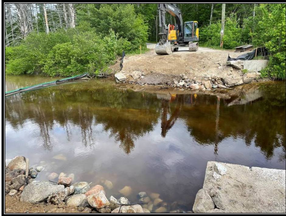
Photo 2: The channel after excavation.
