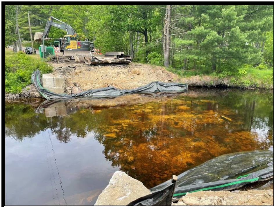
Photo 1: The channel prior to excavation.
