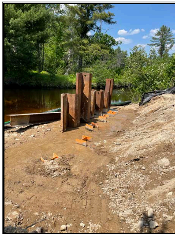
Photo 1: Half of sheet pile sections installed.
