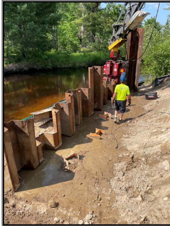
Photo 2: Completed front face of sheet pile sections.
