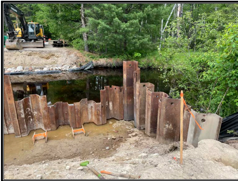
Photo 1: Sheet piles installed on the downstream corner.
