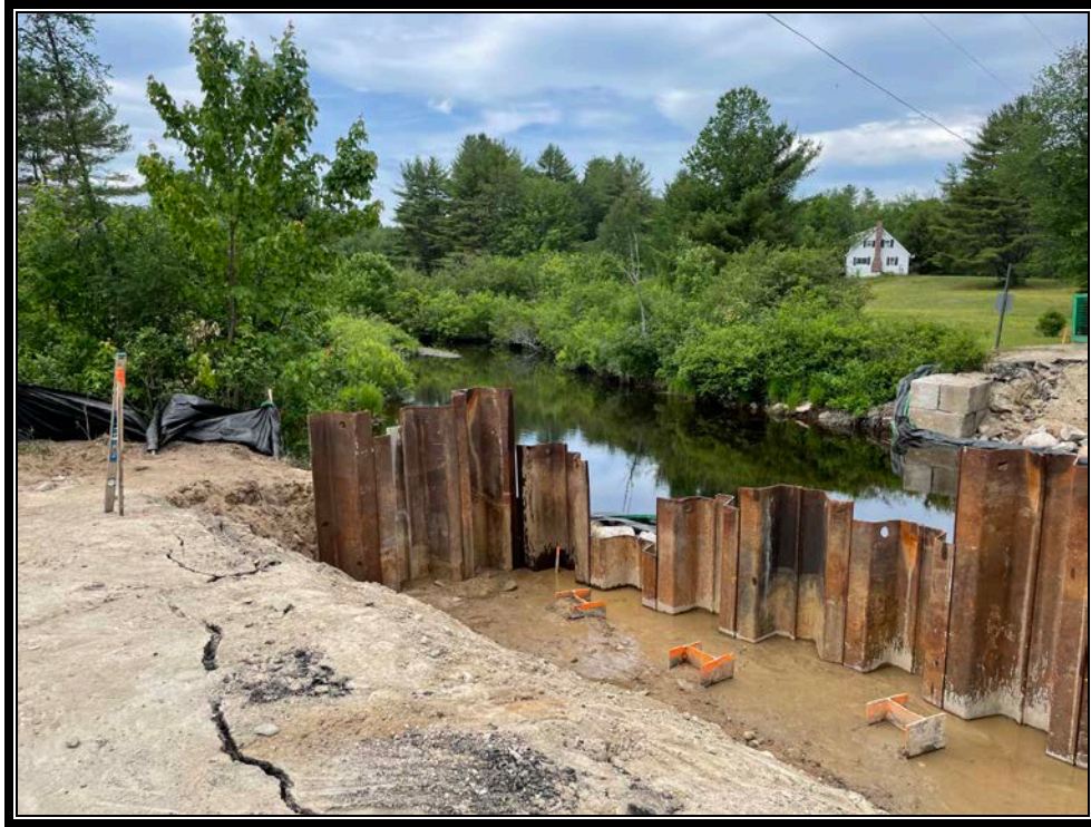
Photo 2: Sheet piles installed on the upstream corner.
