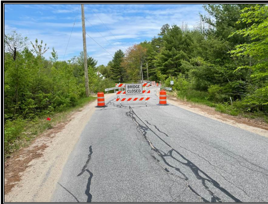
Photo 1: View of bridge closure.
