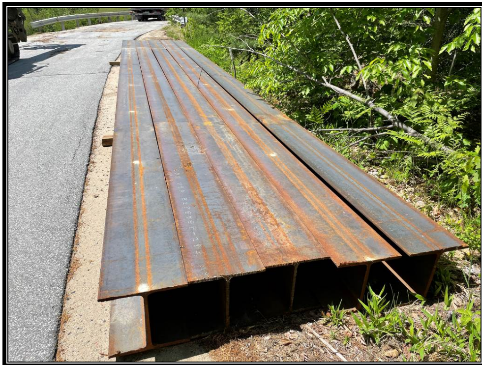
Photo 2: H-Piles delivered to site.
