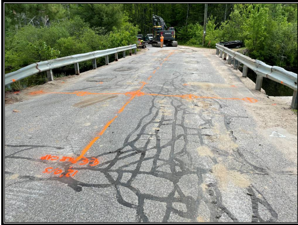
Photo 1: Centerline bearing and pile layout.
