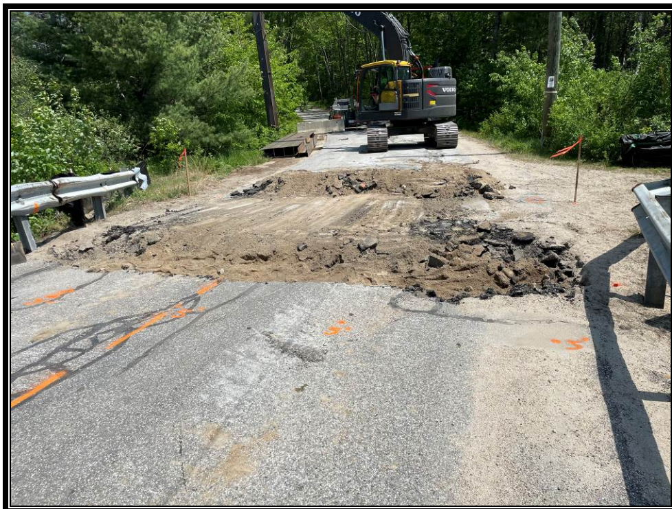
Photo 2: Excavation for piles.
