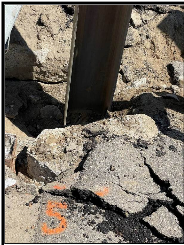
Photo 2: Pile damage repair (P5E).
