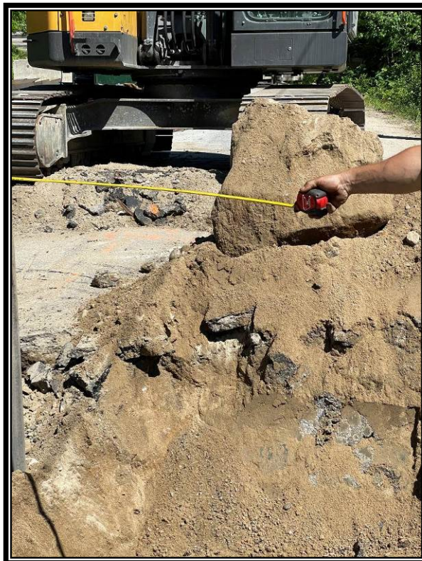
Photo 3: Boulder excavated from P5E pile location.
