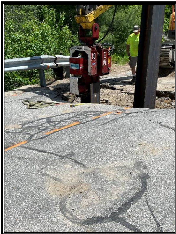
Photo 1: The second H-pile being installed (P4E).
