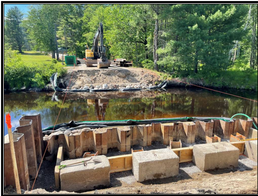
Photo 1: Form mostly installed.
