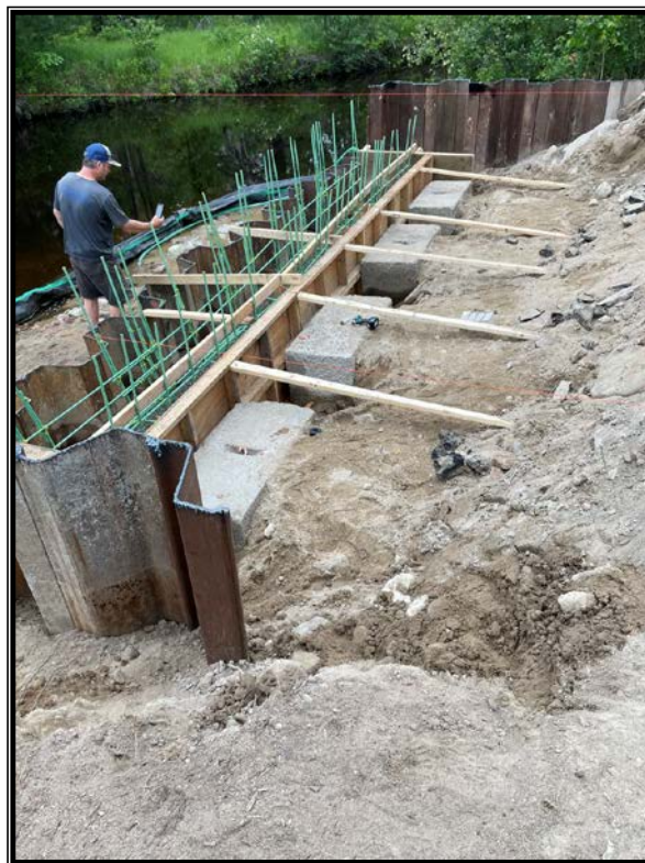
Photo 1: Rebar installed inside forms.
