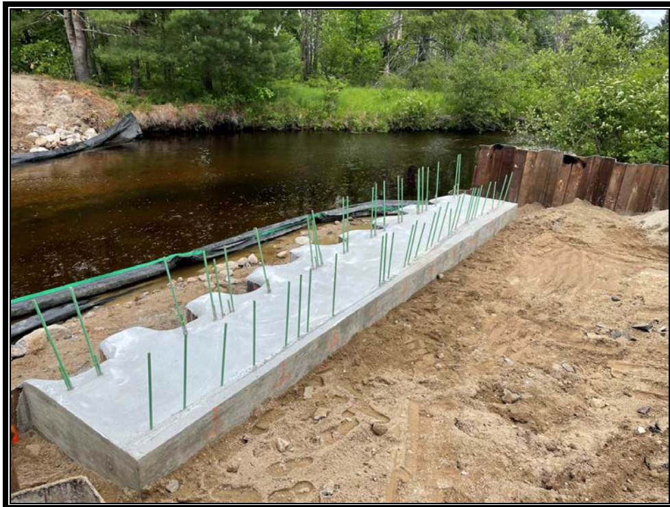
Photo 1: Form stripped off east abutment.
