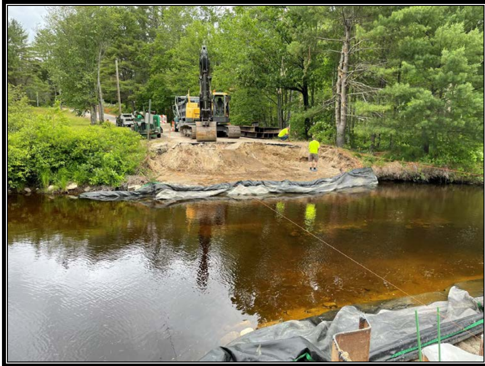
Photo 2: West bank excavated for pile driving.
