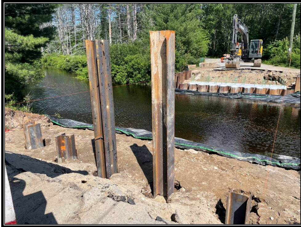
Photo 2: Piles P2W and P3W driven to 27 feet and 28 feet respectively.
