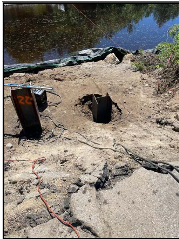
Photo 1: P1W driven to approximately 31 feet.
