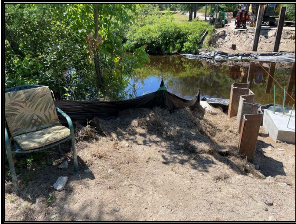
Photo 2: Silt fence maintenance.
