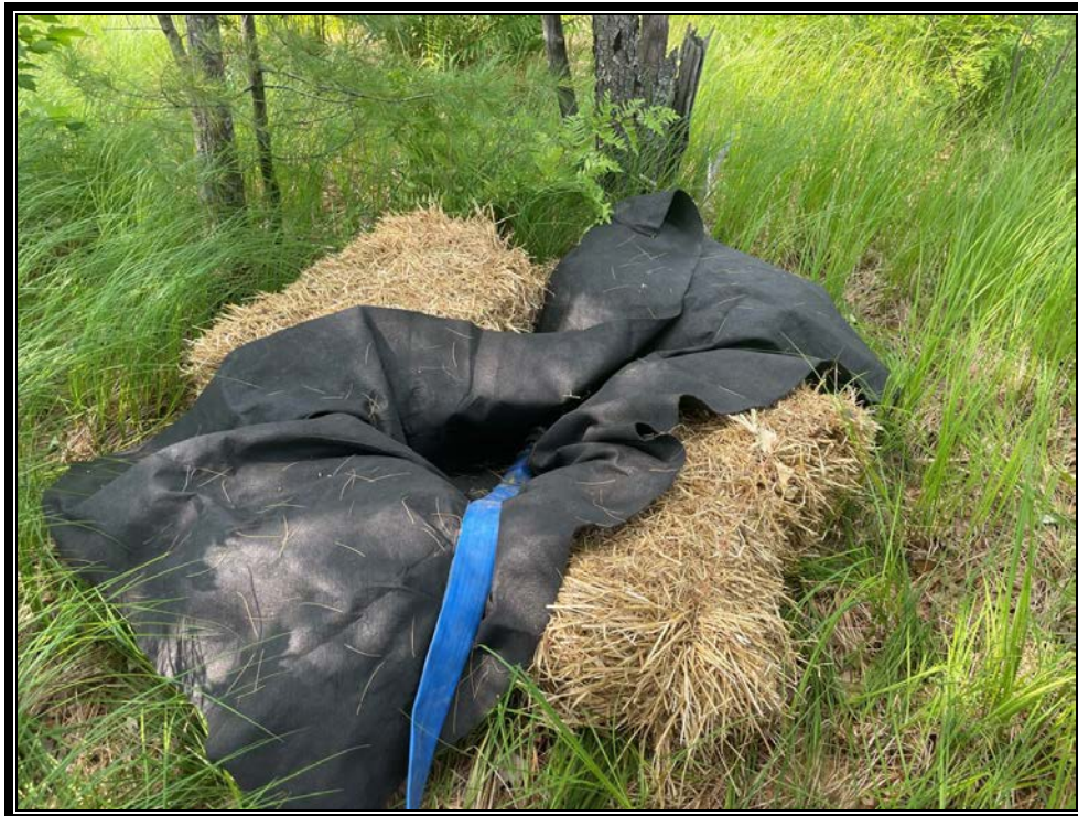
Photo 1: Sedimentation basin on standby for concrete pour.
