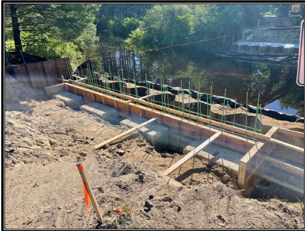
Photo 1: Form and rebar ready for concrete.
