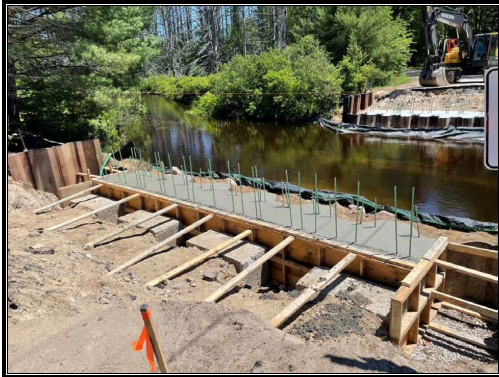
Photo 2: Concrete placed and brought to grade.
