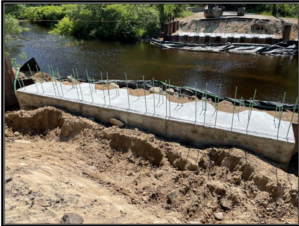
Photo 1: Form removed from west pilecap.
