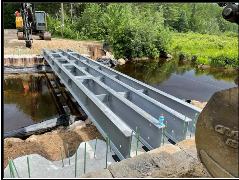
Photo 2: Four out of ten beams placed on bearing pads.
