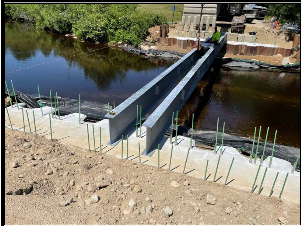
Photo 1: The first two beams being put into rough position.
