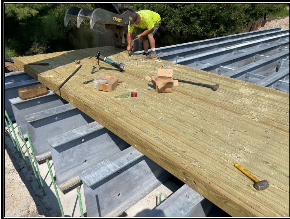
Photo 2: The first two deck sections being secured to the beams.
