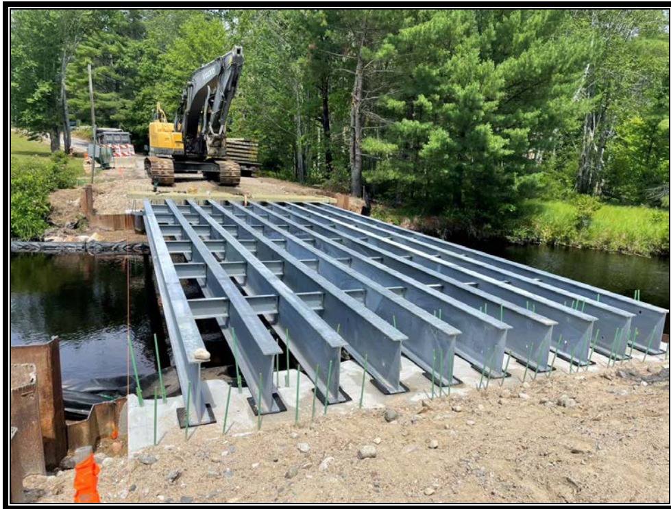
Photo 1: All 10 beams installed.
