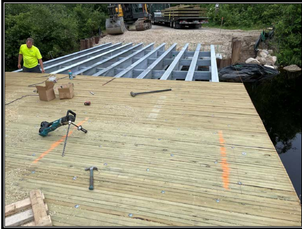
Photo 2: Deck section number 4 being secured to the beams.
