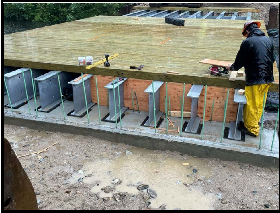
Photo 2: Inside wall of the form being installed.
