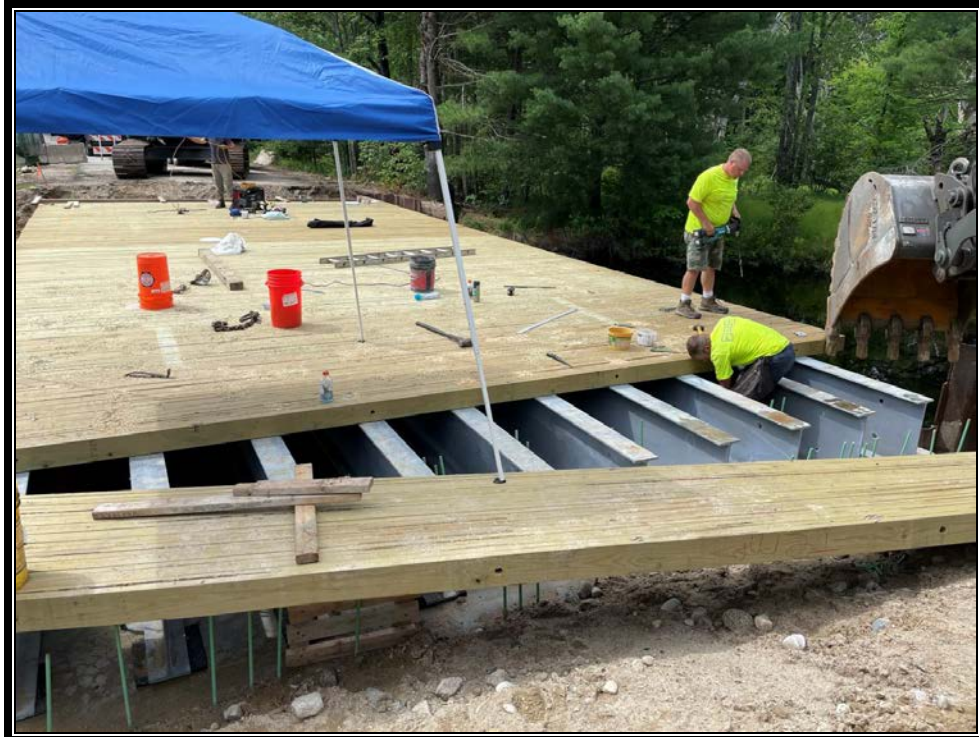
Photo 1: Deck section number 10 being placed into position.
