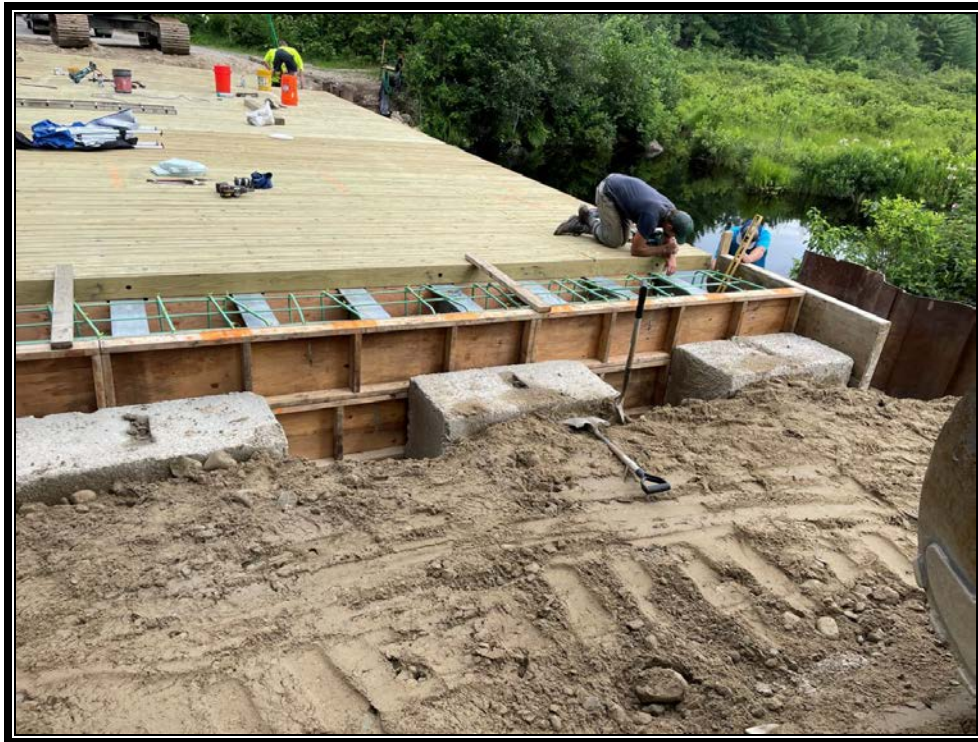
Photo 2: Rebar being placed inside form.
