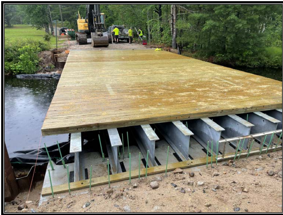
Photo 1: Wooden deck completed.
