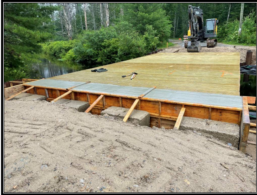
Photo 2: West pilecap second pour completed.
