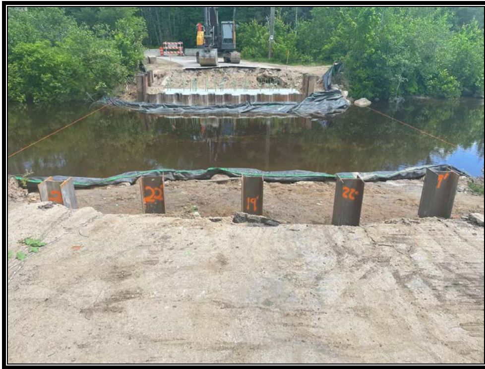
Photo 1: All 5 piles driven to approximately 2/3 intended depth for the day.
