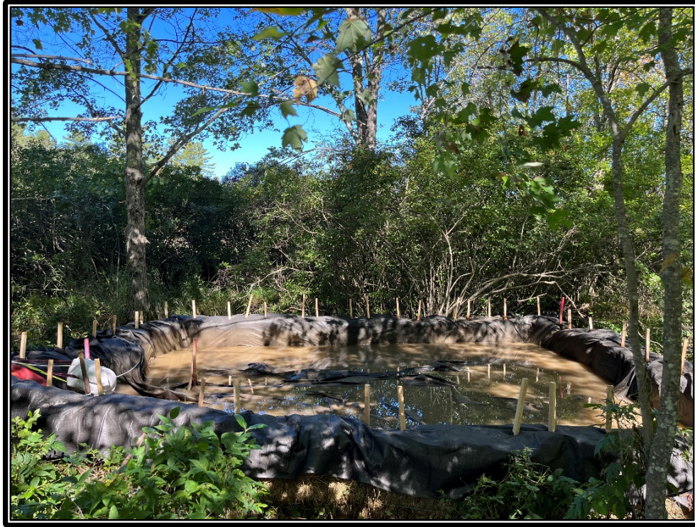
Photo 2: The erosion and sediment control basin constructed on the northeast corner of the site.
