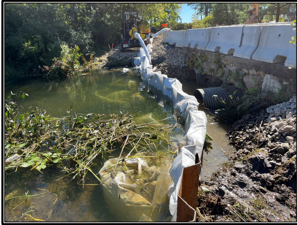
Photo 3: Sheet pile cofferdam with turbidity curtain installed.
