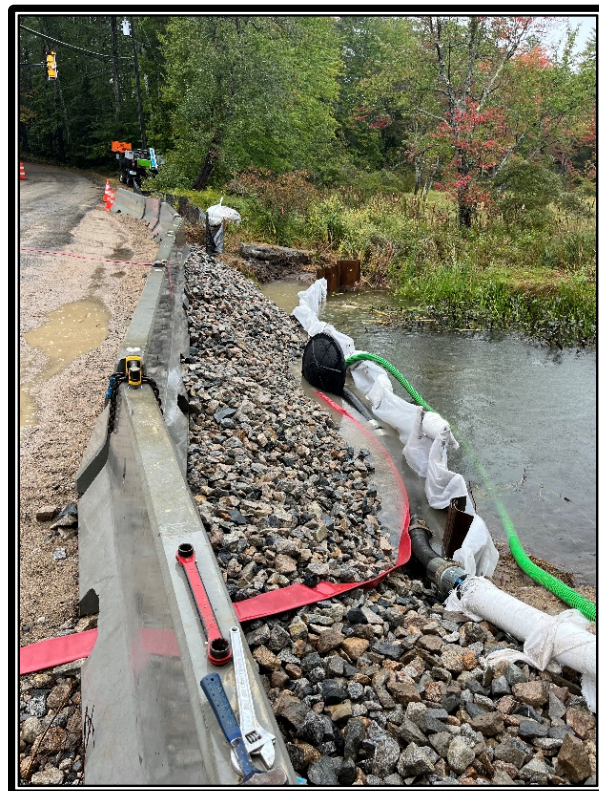
Photo 1: North side of roadway is stabilized with riprap.
