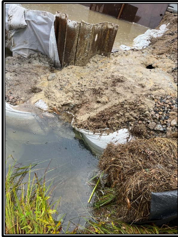
Photo 3: The inlet of the bypass culvert is being held in place by sandbags and roadway material.
