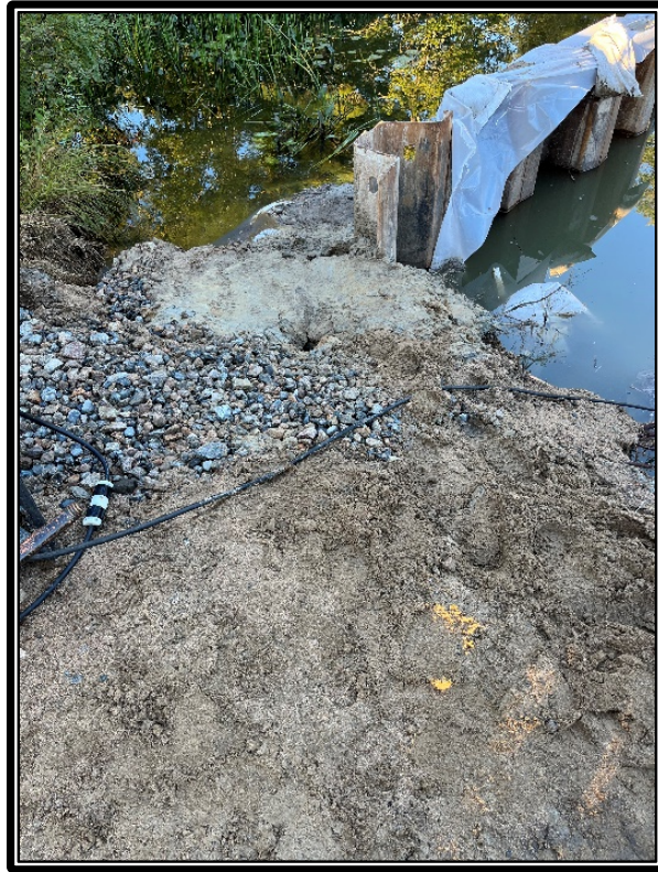
Photo 2: Sinkhole overtop of the bypass culvert.
