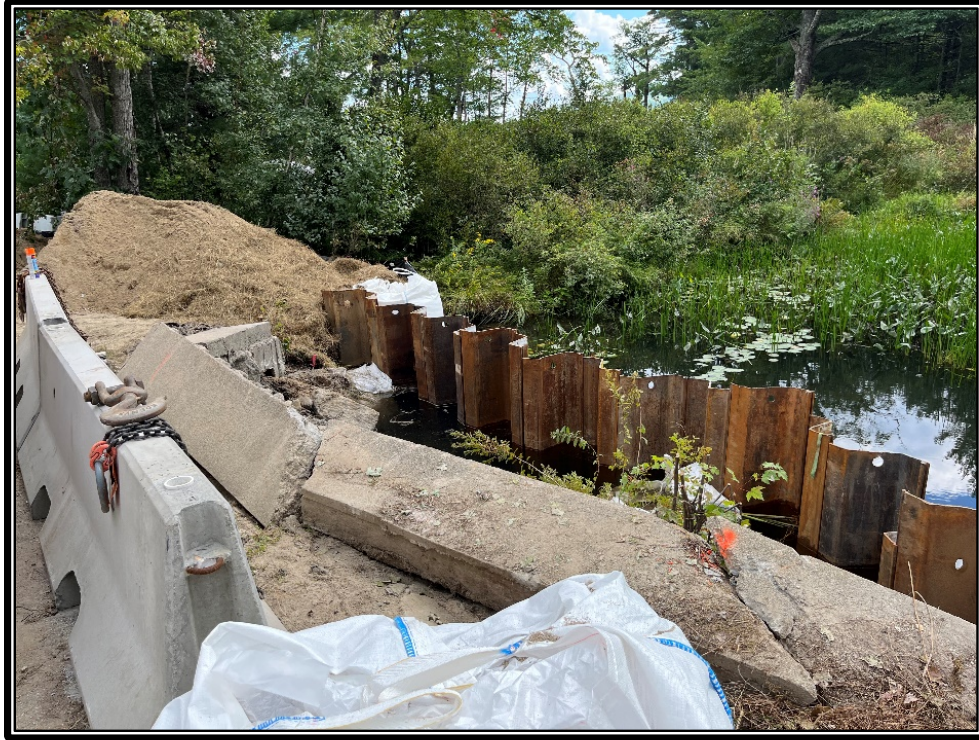
Photo 2: Bridge rail and headwalls were removed. Sheet pile cofferdam nearly complete.
