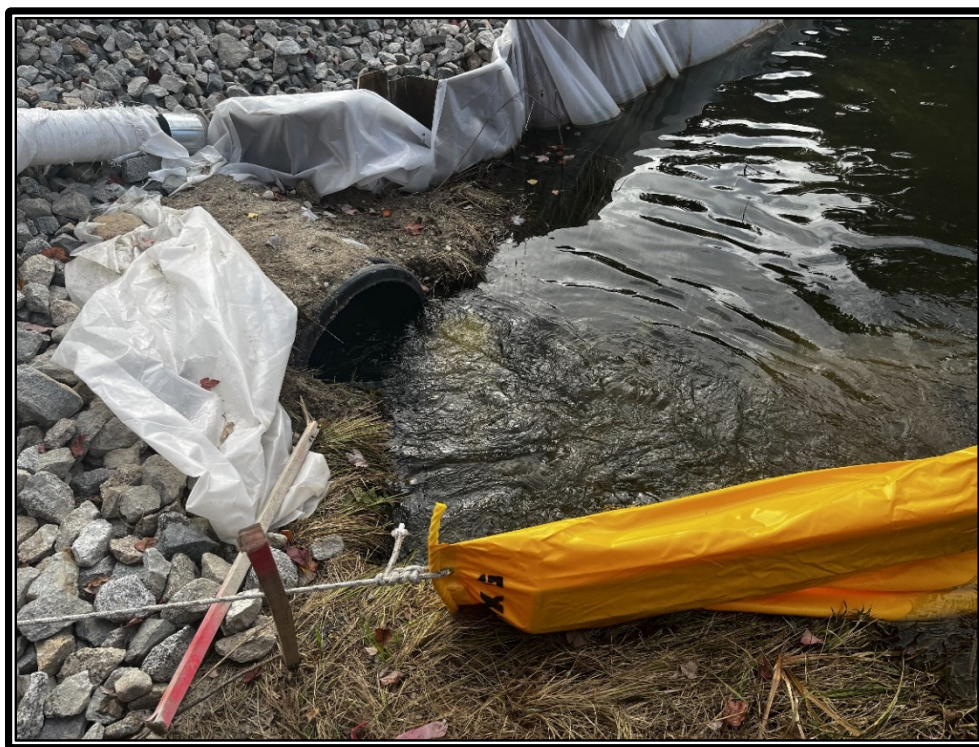
Photo 1: The fill over the bypass culvert at each end remains uncontained by the cofferdam or plastic nor is it stabilized by riprap. The outlet is shown above.
