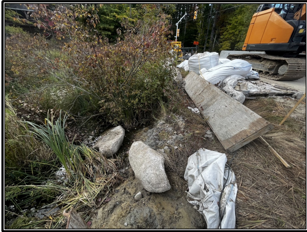
Photo 4: Southwest corner silt fence is missing.
