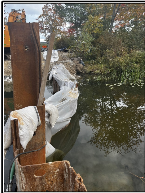
Photo 3: The southeast corner silt fence has been destroyed.
