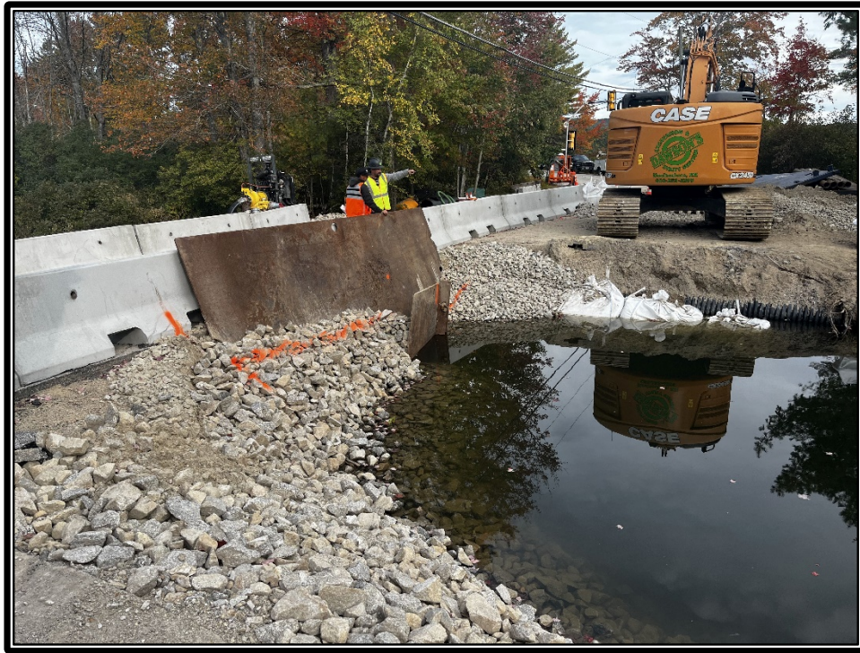
Photo 2: Southern side of roadway being supported by two road plates.
