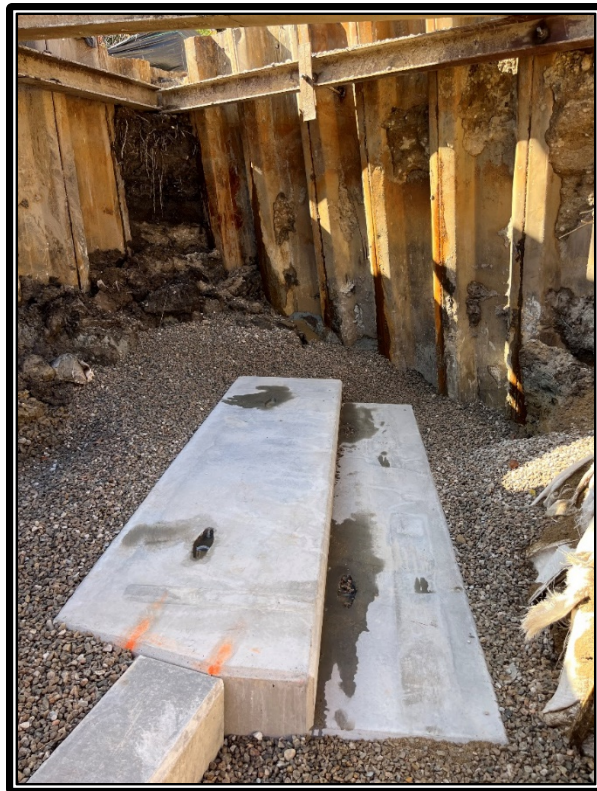
Photo 1: Southwest wingwall footing installed.
