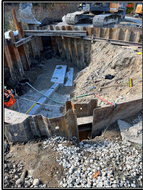
Photo 2: View of Southwest wingwall and cutoff wall from the east side of the excavation.
